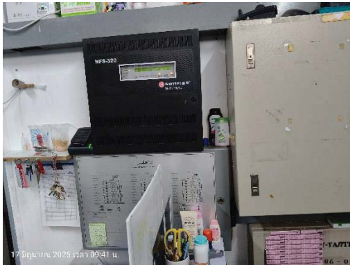
Fire Alarm Control Panel : FCP
